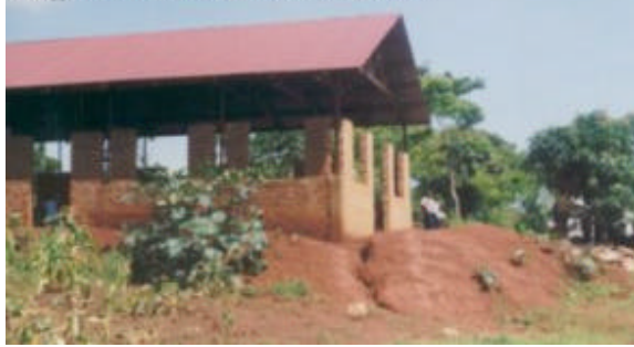
Kajjansi Church construction
